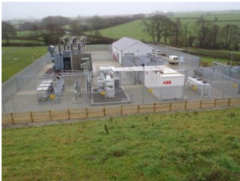
Figure 8: Typical 33/132kV Substation Layout
