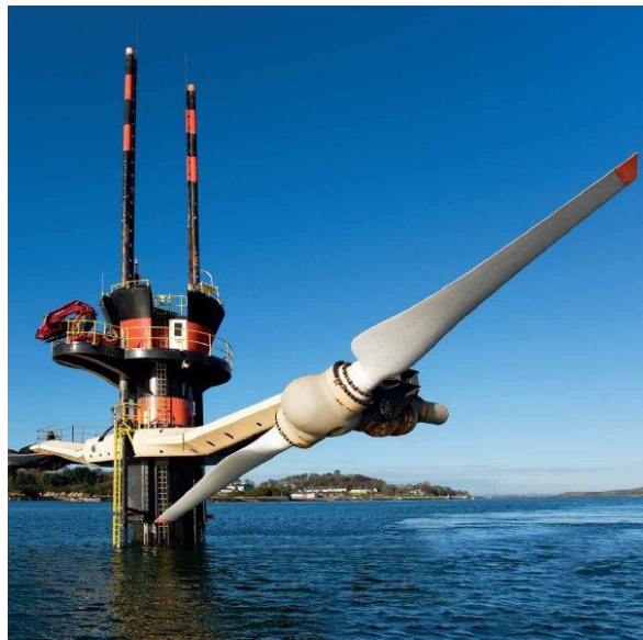
Marine Current Turbines – SeaGen S Mark 2 - (2MW)
