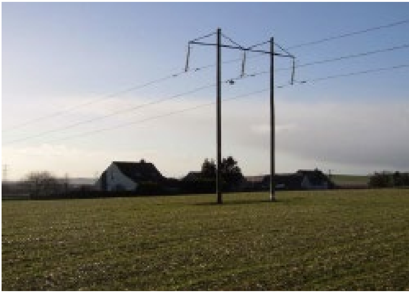
Typical 110kV Wooden Transmission Poles
