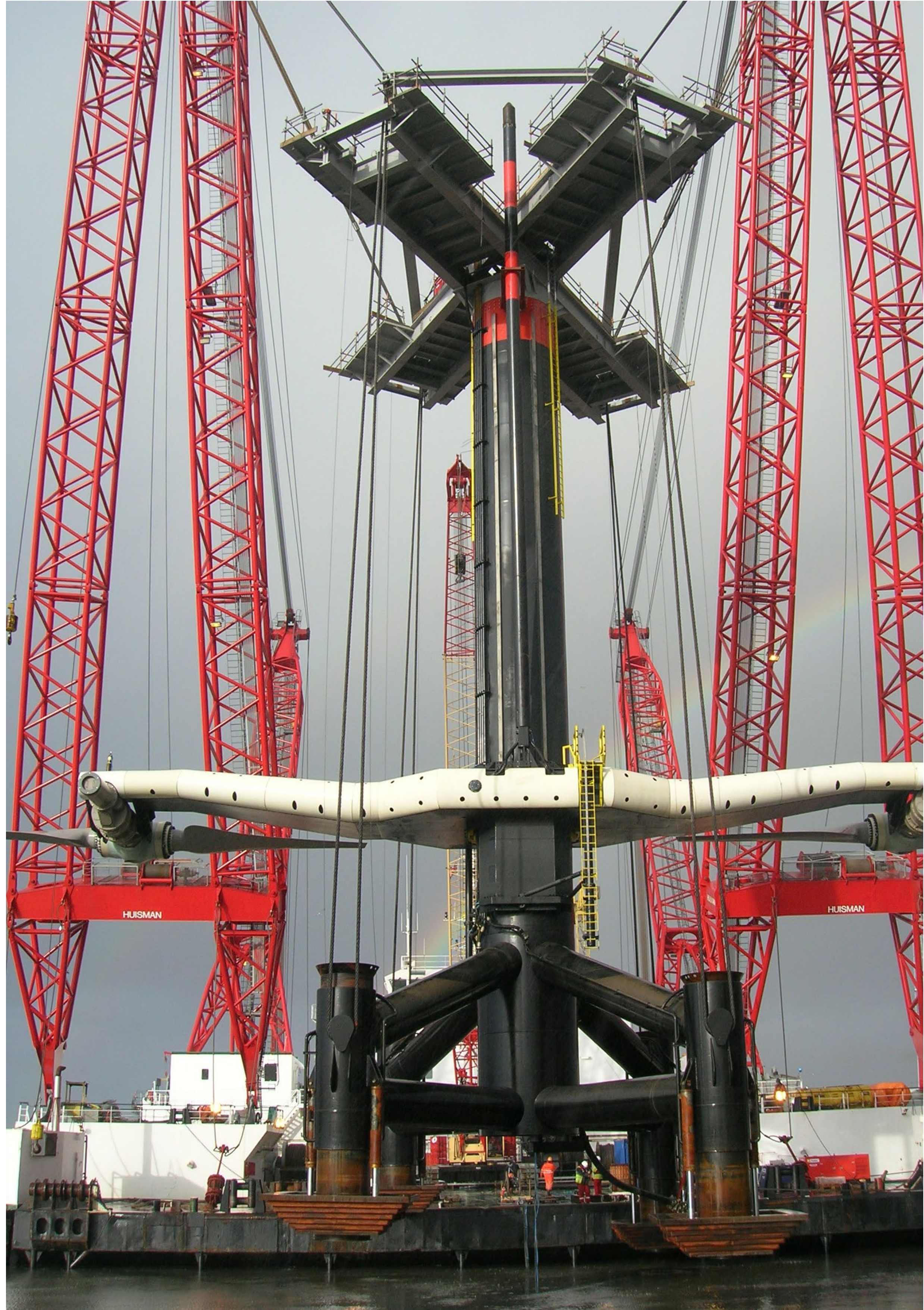
Assembly and loading of SeaGen S at Harland and Wolf Shipyard in Belfast (copyright Harland and Wolf)
